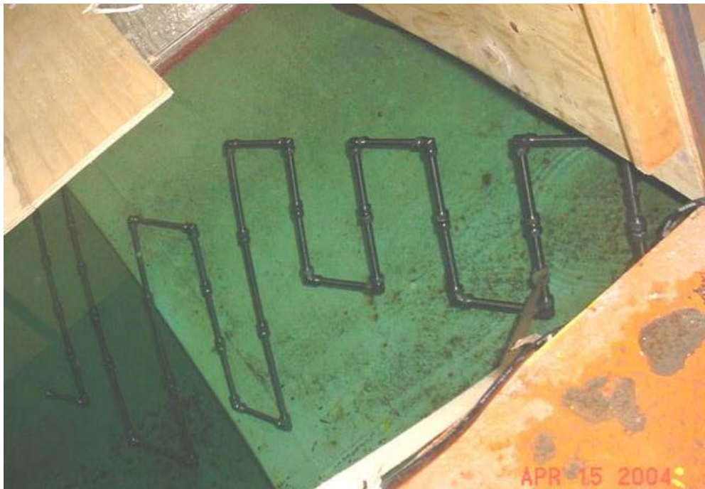
Photograph No. 4. Typical View of Manifold for Pneumatic Proof Test
