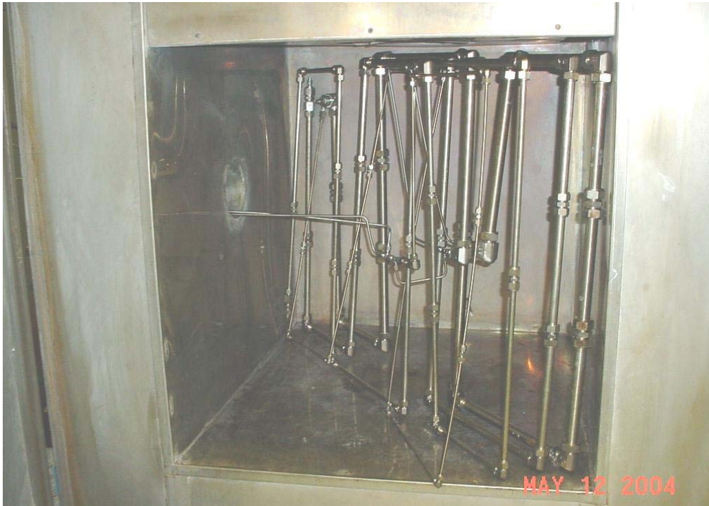
Photograph No. 15. Manifolds Installed in Test Chamber
